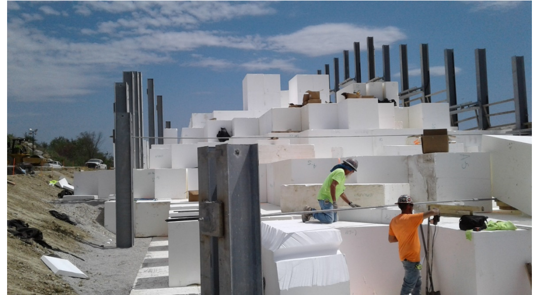
Photo of Yeager Airport Geofoam Wall Construction Photo credit: Schnabel Engineering
