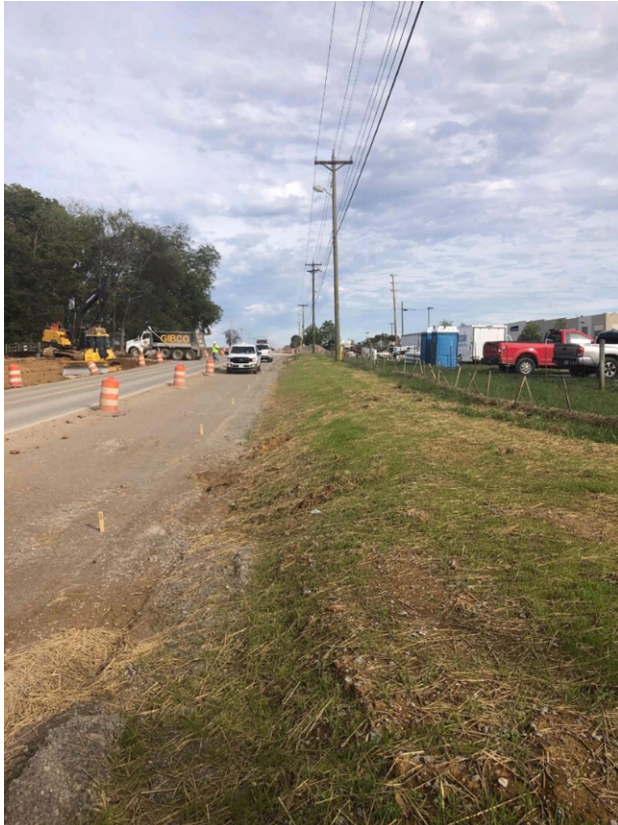
Photograph 1: Base stone Completed from sta. 30 to 50 RT
