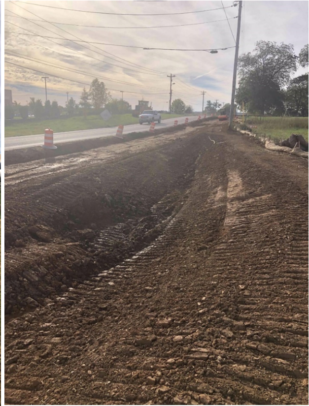
Photograph 2: Grading of ditches near Private Drive 1
