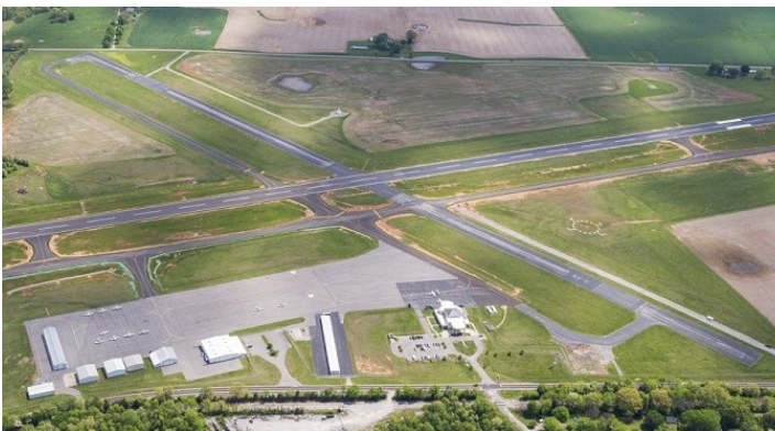
Outlaw Field Airport in Clarksville, TN after Major Reconstruction of the Primary Runway and Taxiway
