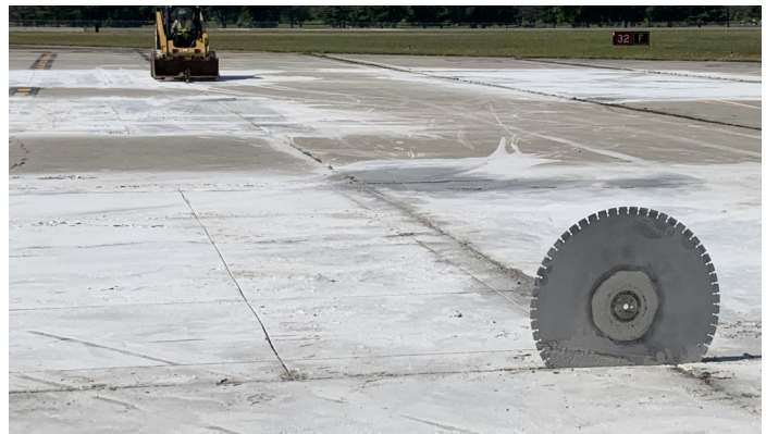
Smyrna Airport in Smyrna, TN during Taxiway Foxtrot Hold Pad Repair
