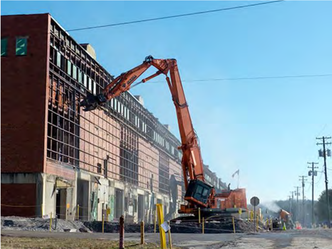
Demolition of Building K-27 Begins (DOE photo)
