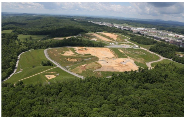
The Y-12 chestnut ridge non-hazardous waste disposal facilities left, and nonhazardous demolition activities above. (DOE Photos)
