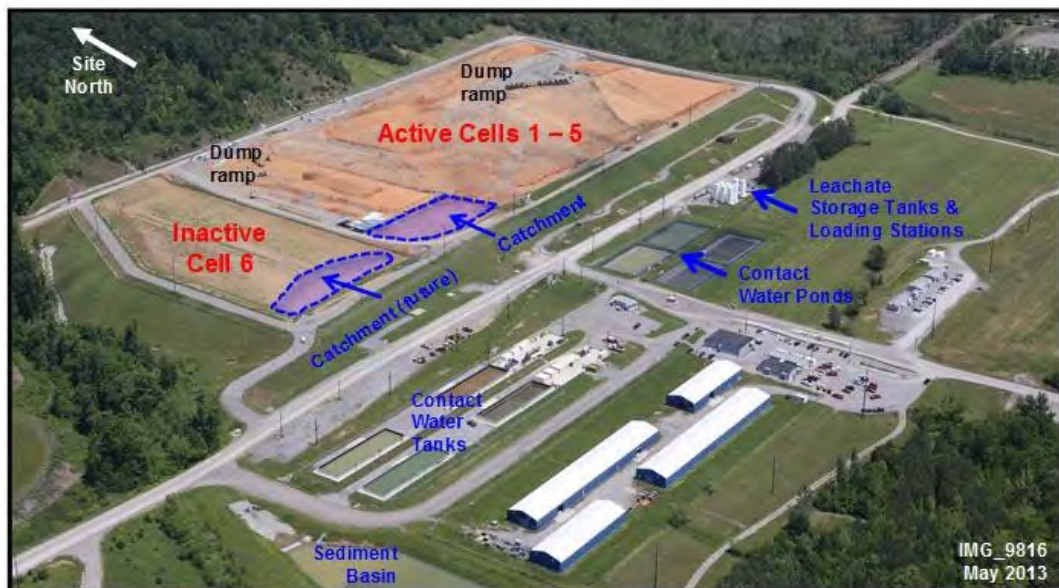
Fig. 3. Environmental Management Waste Management Facility.
