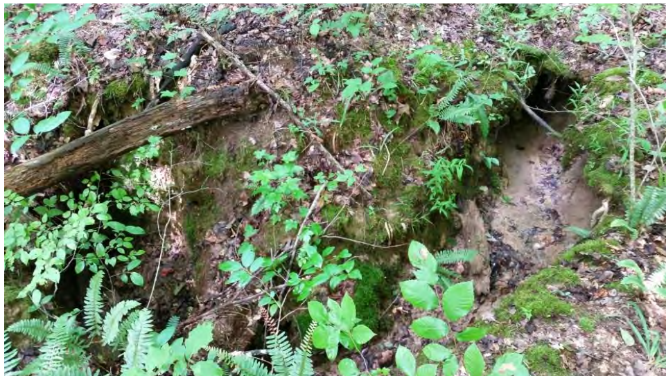
Fig. 11. Headwater soil channel daylighting point.
