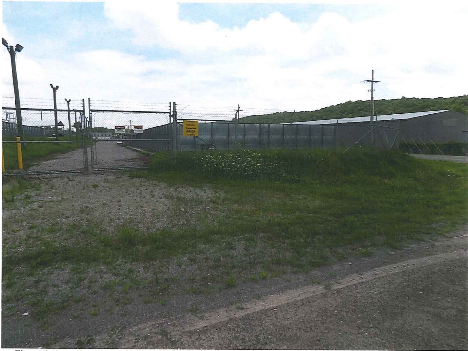
Figure 6. Fenced contact water tanks at the Environmental Management Waste Management Facility (EMWMF).
