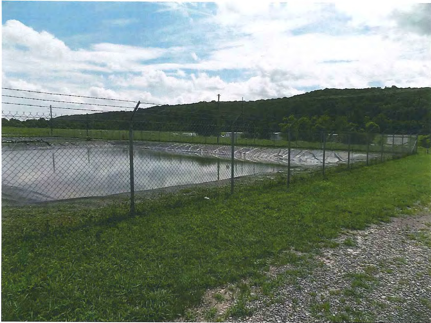
Figure 5. Fenced contact water ponds at the Environmental Management Waste Management Facility (EMWMF).
