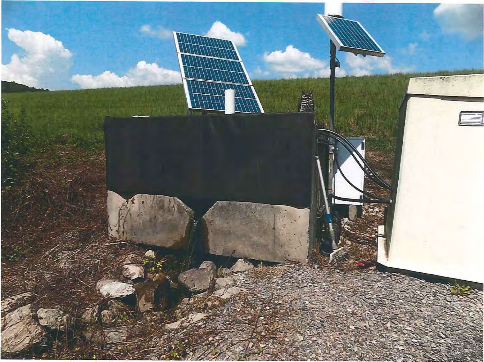
Figure 7. Environmental Management Waste Management Facility (EMWMF) V-weir.
