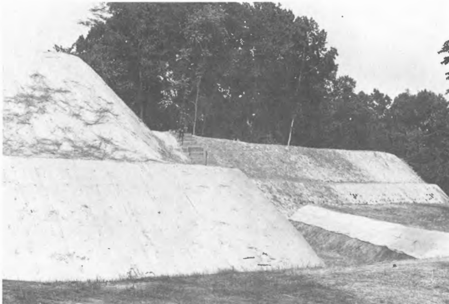
FIGURE 9: Union fort during restoration (top), exterior parapet and moat after restoration (bottom)
