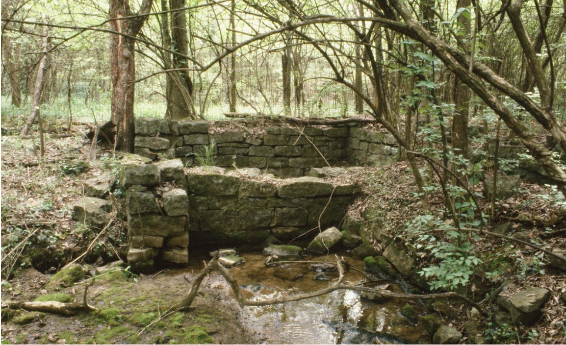
Figure 25. Remnant East Tract springhouse (facing east).
