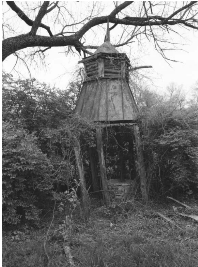
Figure 26. Cupola over a West Tract sulfur well (facing southeast).
