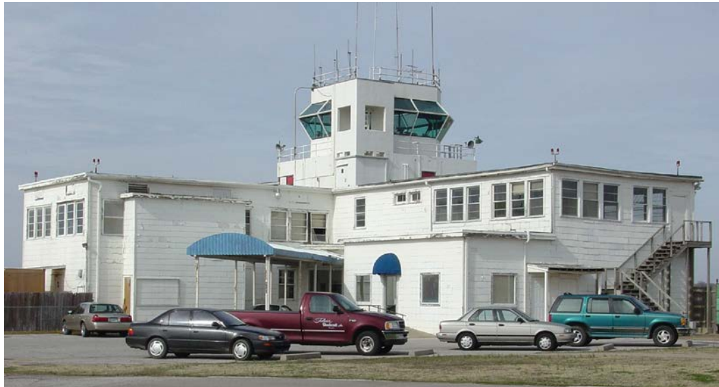
Figure 15. 2006 photo of World War II era control tower at the former Memphis Naval Air Station. (TDOA WWII image file, photo #138a).
