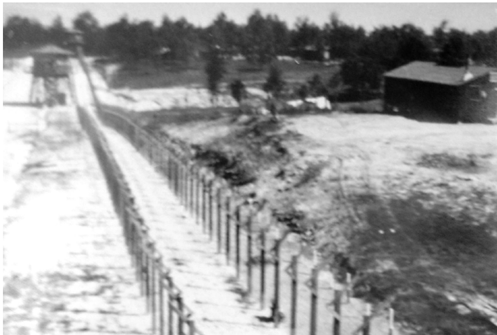
Figure 10. Perimeter fence for prisoner compound at Camp Crossville. Guard tower is in background with barracks at right (copied from original photo housed at University of Tennessee Agricultural Extension Service 4-H Camp, Crossville).
