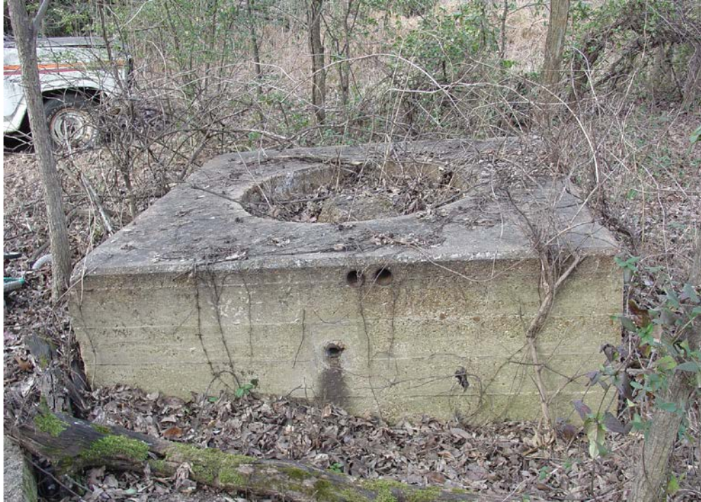
Figure 25. Concrete structure for anti-aircraft gun turret at 40LA174 (TDOA WWII image file, photo #S046).
